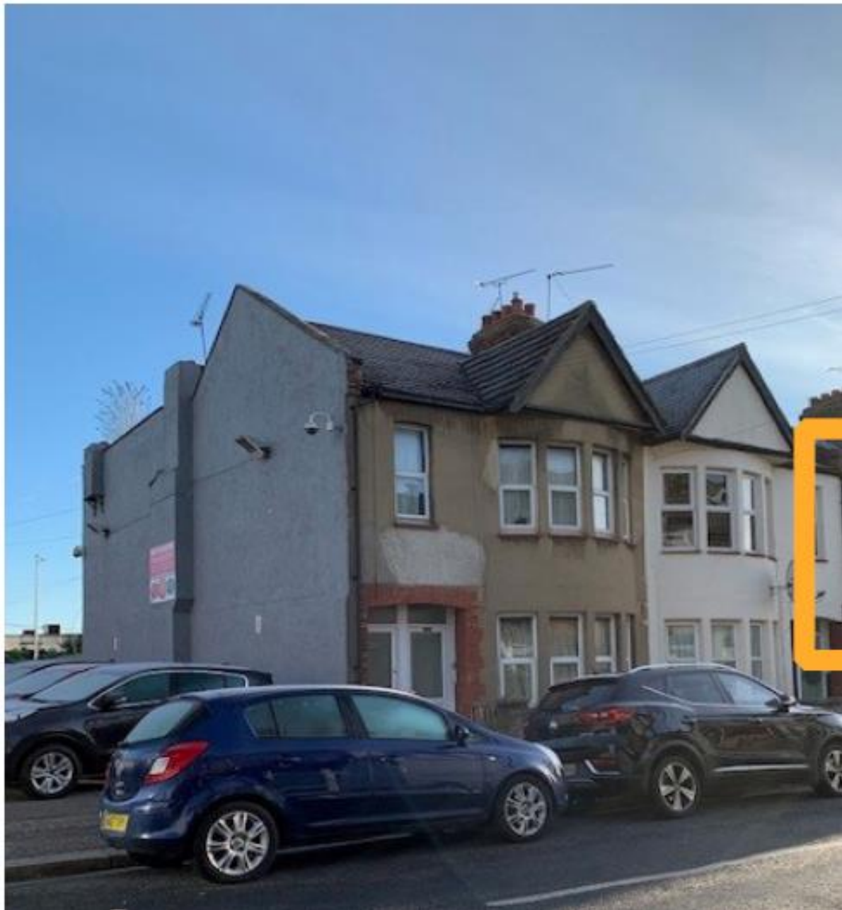
View to No's 10 & 12 Chase Road
